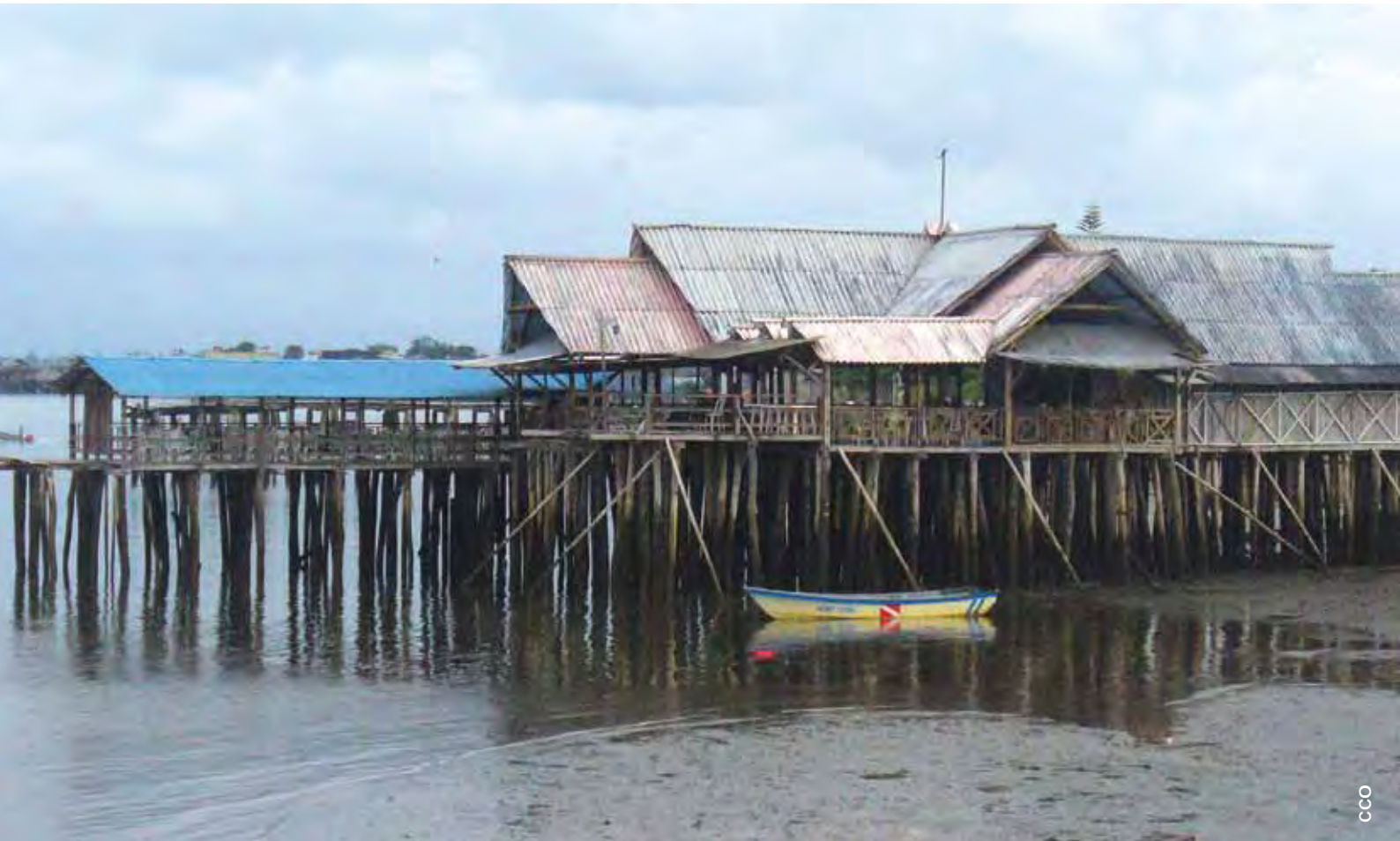
Construction sector of pile-dwelling in Tumaco.
