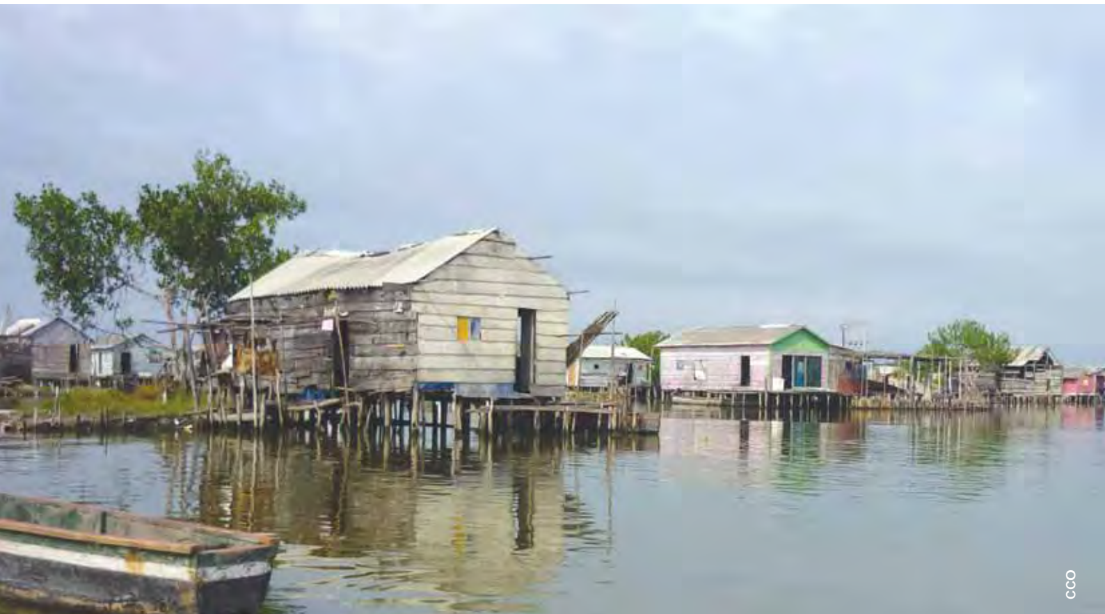
Construction sector of pile-dwelling in Tumaco.
